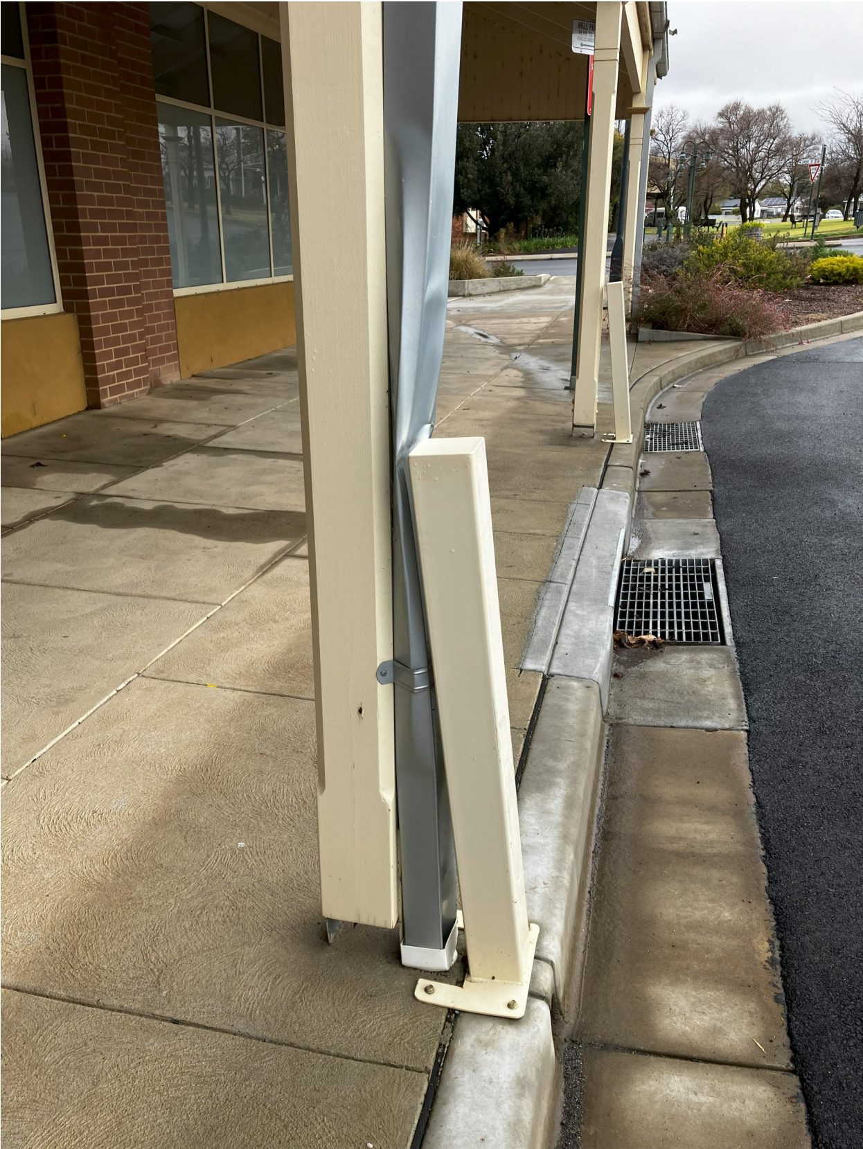
Damage to posts with 300-450 mm setback Main Street Medical
